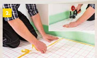
Fix the edge insulation strip to the Velcro system roll using the adhesive strip (or adhesive tape at the ends)
