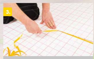
Use the adhesive strip to connect the Velcro system rolls at the foil overlap at the sides
