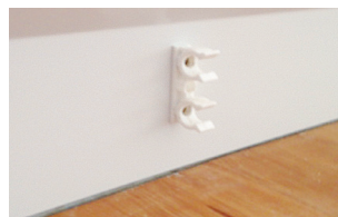
Installation of pipe clip
