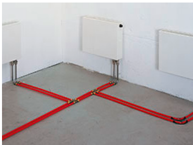
Radiator connection from the floor
